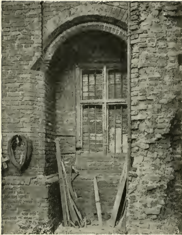
(a) ARCH UNDER CHIMNEY-STACK
